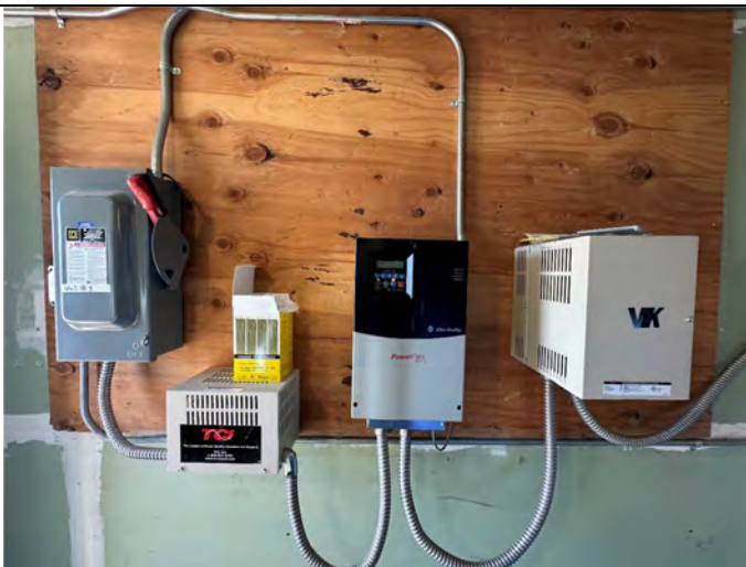
PHOTOGRAPH 7 Current electrical configuration for irrigation supply.
